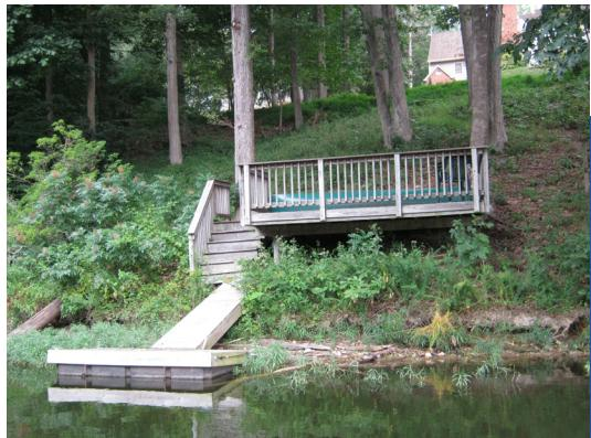
**Pier/Float Combination:** A floating dock connected securely to a pier.
