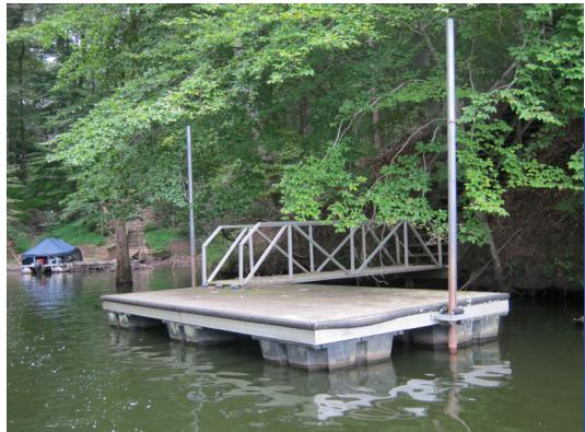
**Float:** A platform which floats on the surface of the water and is securely attached to either the shore or to a pier.
